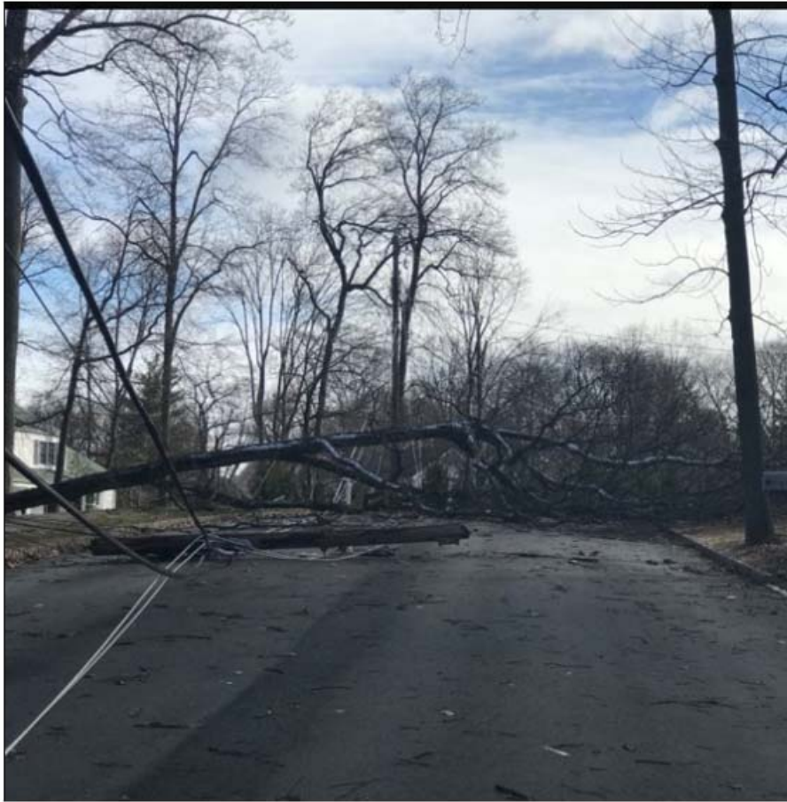
March Winter Storm Damage in Basking Ridge
